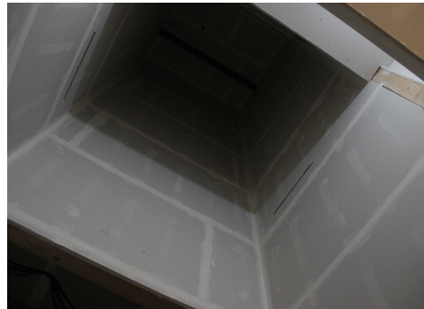
Elevator shaft is complete... elevator coming soon
