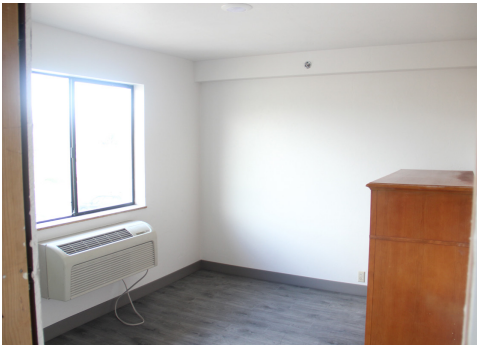
New flooring installed in guest rooms and staff offices
