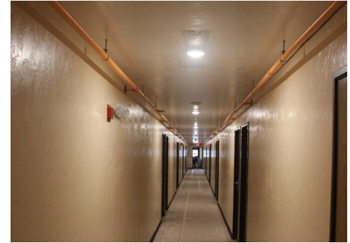
2nd floor fire suppression system underway
