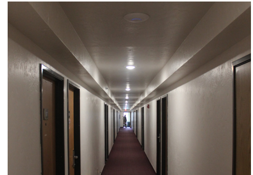
3rd floor fire suppression system completed
